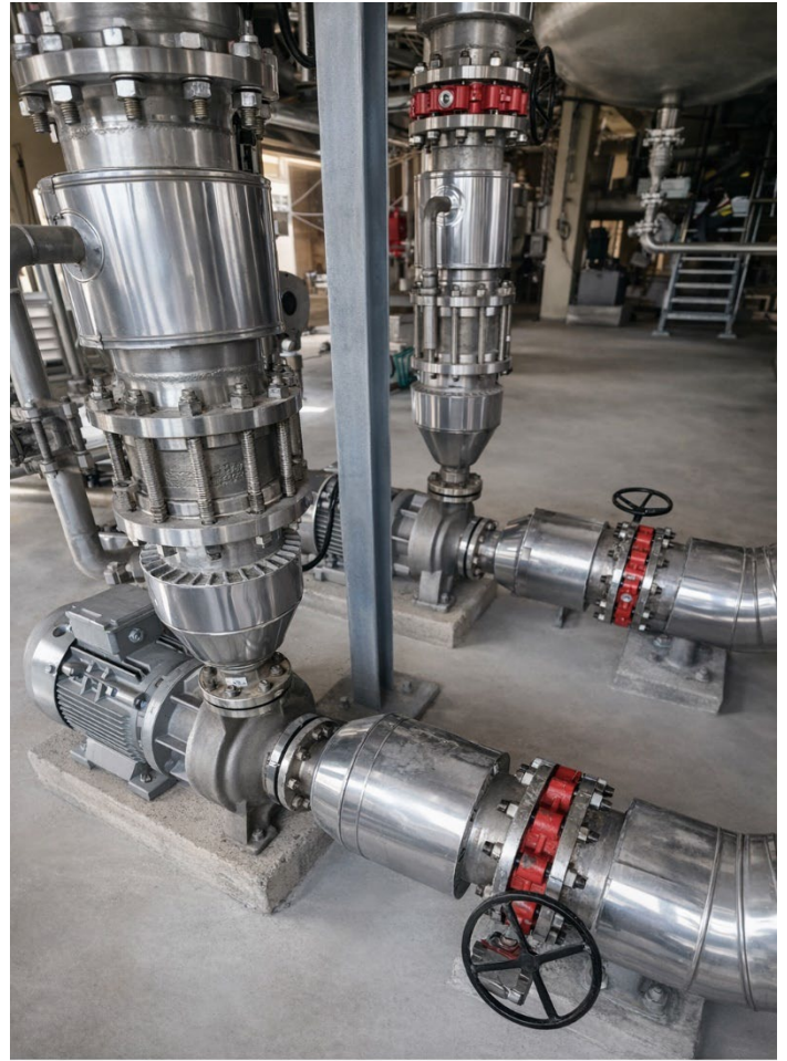
Cooling water system installation – data center project (Sweden)
